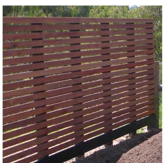
Timber slat screen fence
