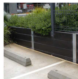
Coloured Concrete Sleeper Retaining Wall
